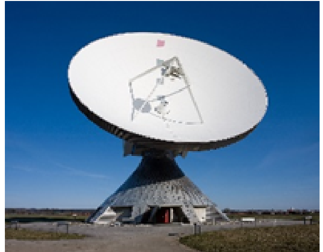
Radar Tracking System
